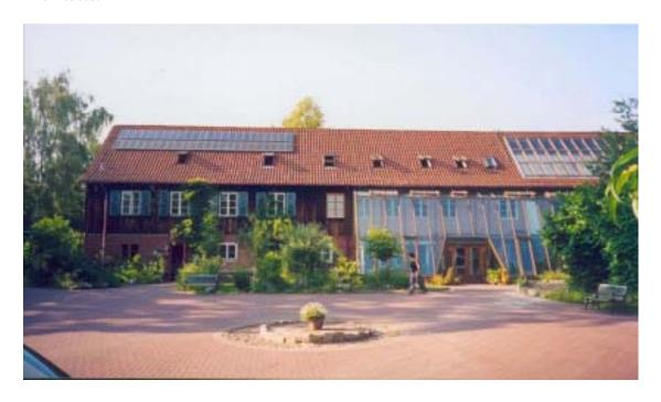
The 60 house eco-village of Lebensgarten at Steyerberg in North Germany has a fully integrated energy policy which includes a Combined Heat and power plant for on-site electricity and district heating. It is supplemented by both thermal and photovoltaic solar energy systems.
