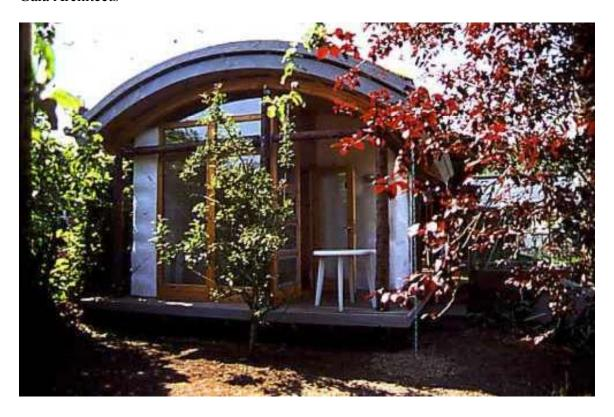
A client with an experimental nature helped this innovative project to become reality. The frame is of roundpole, the walls of straw rendered on both sides with lime plaster. The sheep wool insulated roof was covered with turf.
