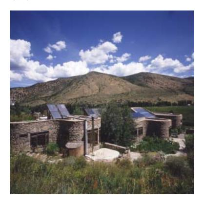
Situated at 2200m above sea level, outdoor temperatures during the winter can fall to -44°C. Blizzards are common. 1% of the heating needs of the building are provided by two small wood burning stoves and 99% from passive solar. Conventional heating is not needed. The heavy thermal mass curved building stores heat and a large glazed south facing façade allows three-quarters of the light and half of the solar energy to enter the building and retains it.
