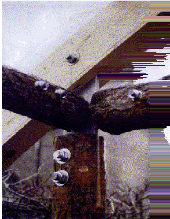
Fig. INFRA 6 Roundpole Connection using Galvanised steel pieces at Raymond's Smoke Shed in Dunning, Perthshire
